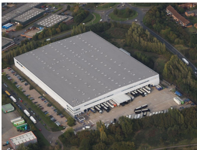
House of Fraser National Distribution Centre Wellingborough
